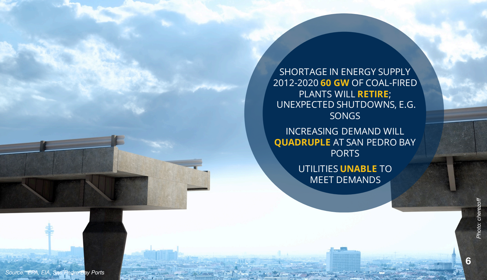
Source: EPA, DOT, The White House
